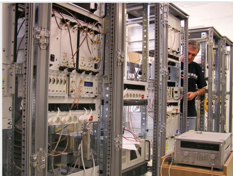
Road Tunnel Technology Assembling
