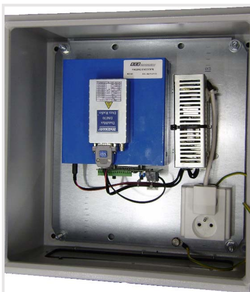
Paging base equipment with encoder and power supply
